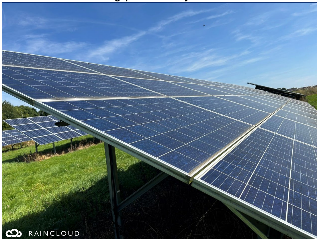
Plate A9.1.18: Rainwater gaps on PV array table
