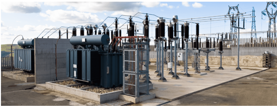
Plate A9.1.10: Typical substation connection arrangement
